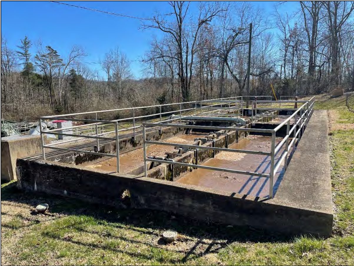
Figure 5.3.1 Aerobic Digester
