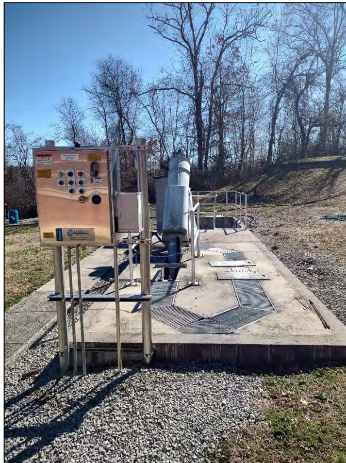
Figure 5.2.1 Mechanical Screen
